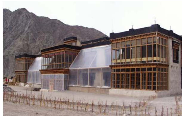
Fig. 9: SECMOL training Centre – Ladakh, showing passive design for minimum energy demand. (Source: SECMOL. http://www.secmol.org/solarenergy/ )
